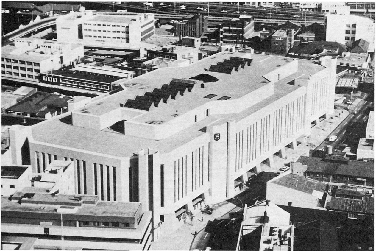
Fig. 2. The Standard Bank Administration Building
