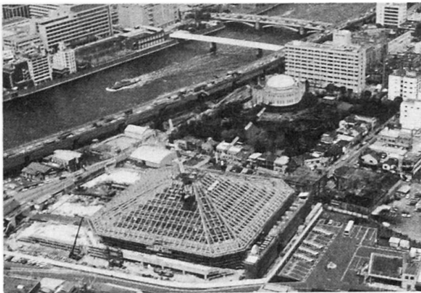
Space frame under construction
