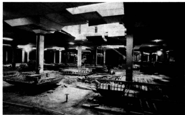
Figure 4 Floor B1 under construction
