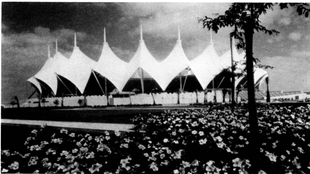
Fig. 7: Roof after Completion
