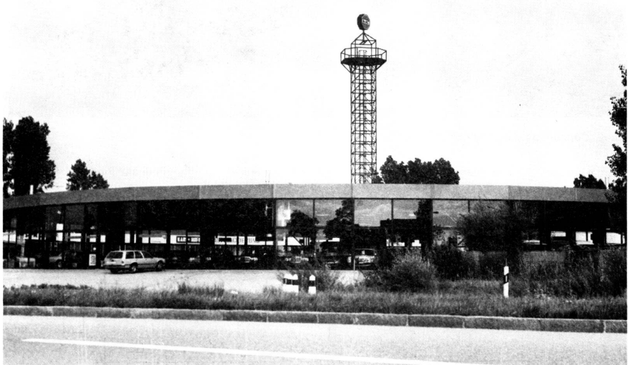
Fig. 1 Outside view of the hall
