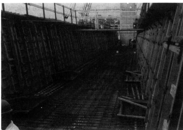
Fig. 4: After placing of inner web formwork
