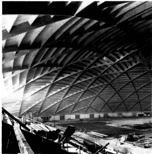
Inside view of the dome after erection
