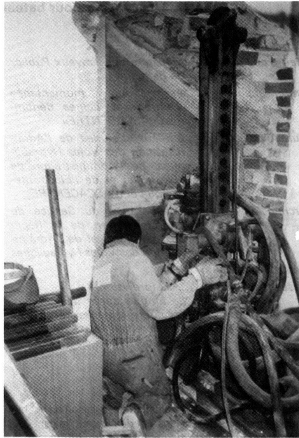
Fig. 2 Through excavations in the supportive brick walls holes were sunk vertically through the basement walls.
