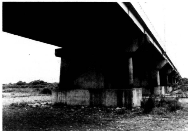
Fig. 7 After repair (Natori Bridge)
