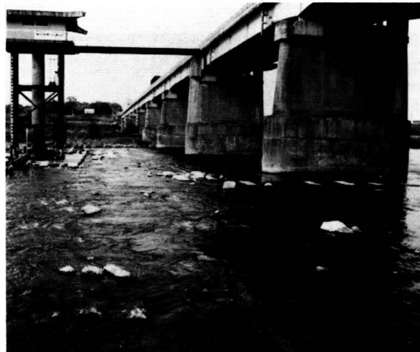
Fig. 3 After repair (Iwaide Bridge)
