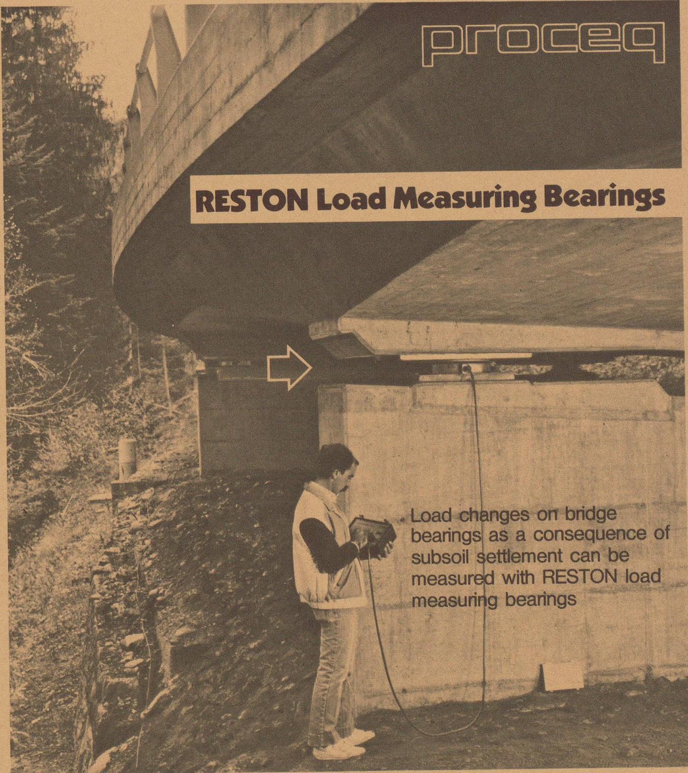
Load changes on bridge bearings as a consequence of subsoil settlement can be measured with RESTON load measuring bearings
