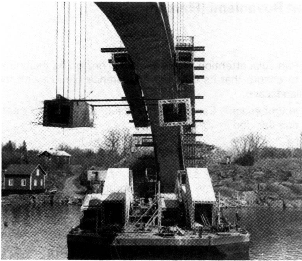
Fig. 4 Erection of the arch elements
