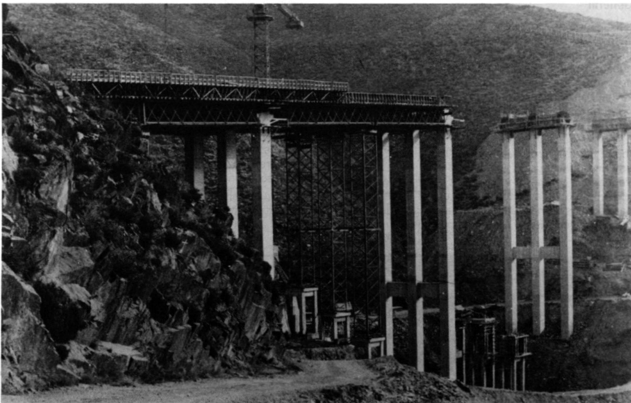
Fig. 3 Site construction works
