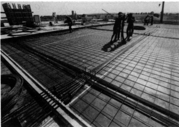
Fig. 5 Placing of VSL Monostrand tendons for the roof post-tensioning
