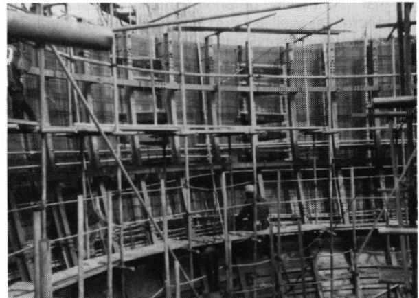
Fig. 3 View of the formwork; note the block-out forms for the horizontal post-tensioning
