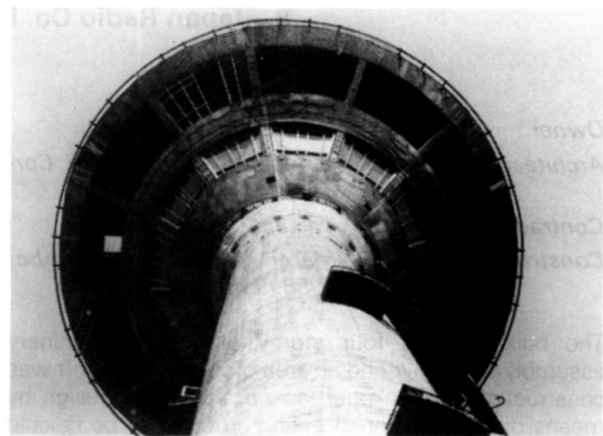
Fig. 3 Bottom view of skypod floor
