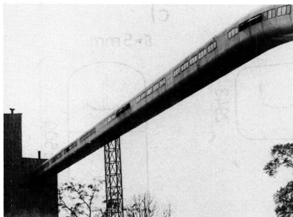
Fig. 5 General view of a gallery situated: a) in straight line, b) in broken line
