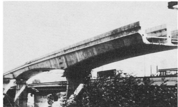
Photo 2 - Clichy bridge. General view of a pier-head beam.
