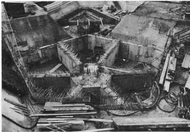
Fig. 9: Cellular foundation under one of the main columns
