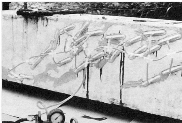
Fig. 18 Example of Crack Grouting
