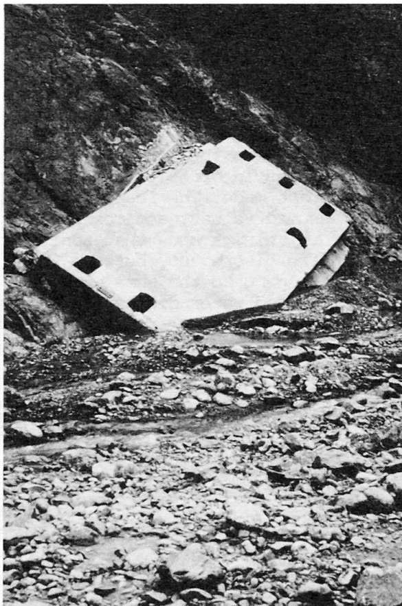
FIG. 2 200 Ton Bridge slab after the flash flood.
