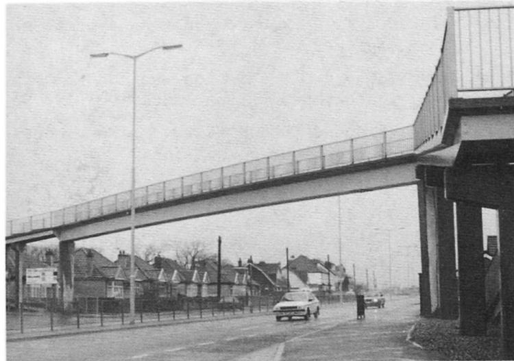
Fig.8 Stoke Lane footbridge
