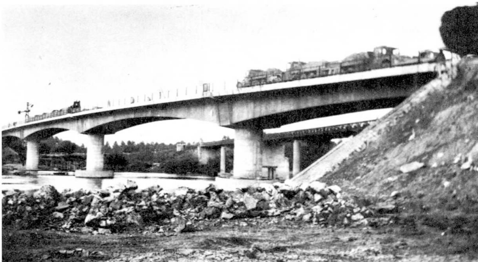
Fig.1 The 5-span bridge concreted without falsework across the river Váh at Kollárovo during testing
