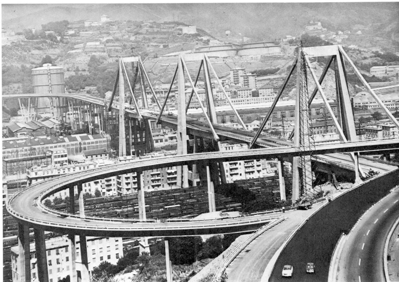
Figure 3 - General view of the structure.
