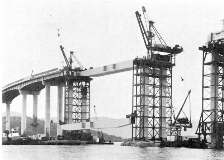
Fig. 11 Box girder erection
