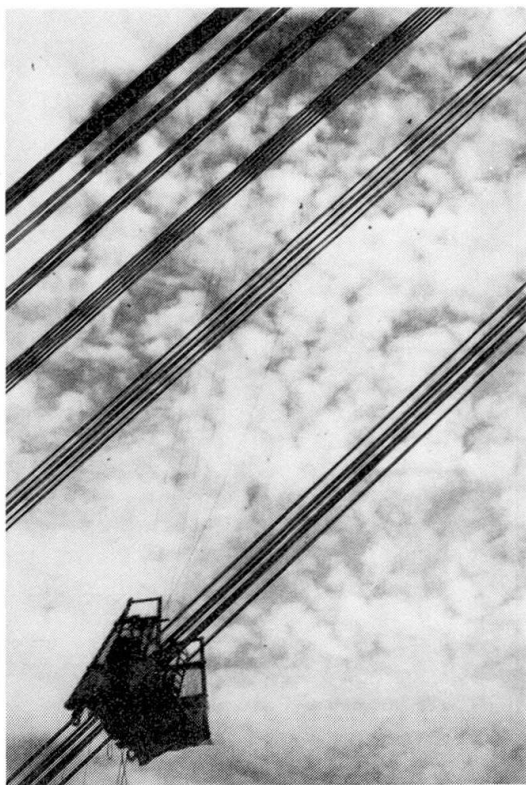
Fig. 10 Inspection of Cables
