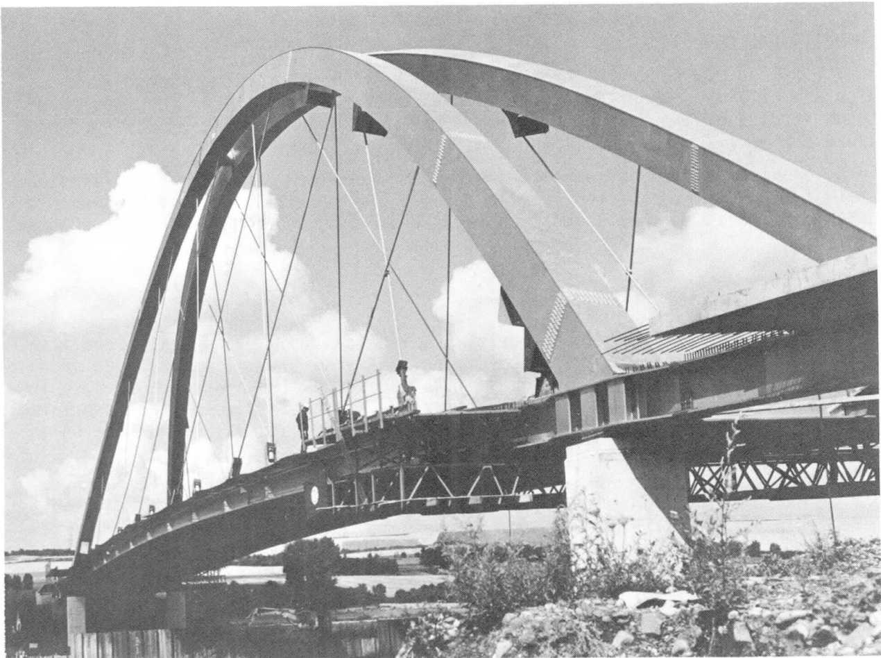
Fig. 10 Bridge at Hermalle.
