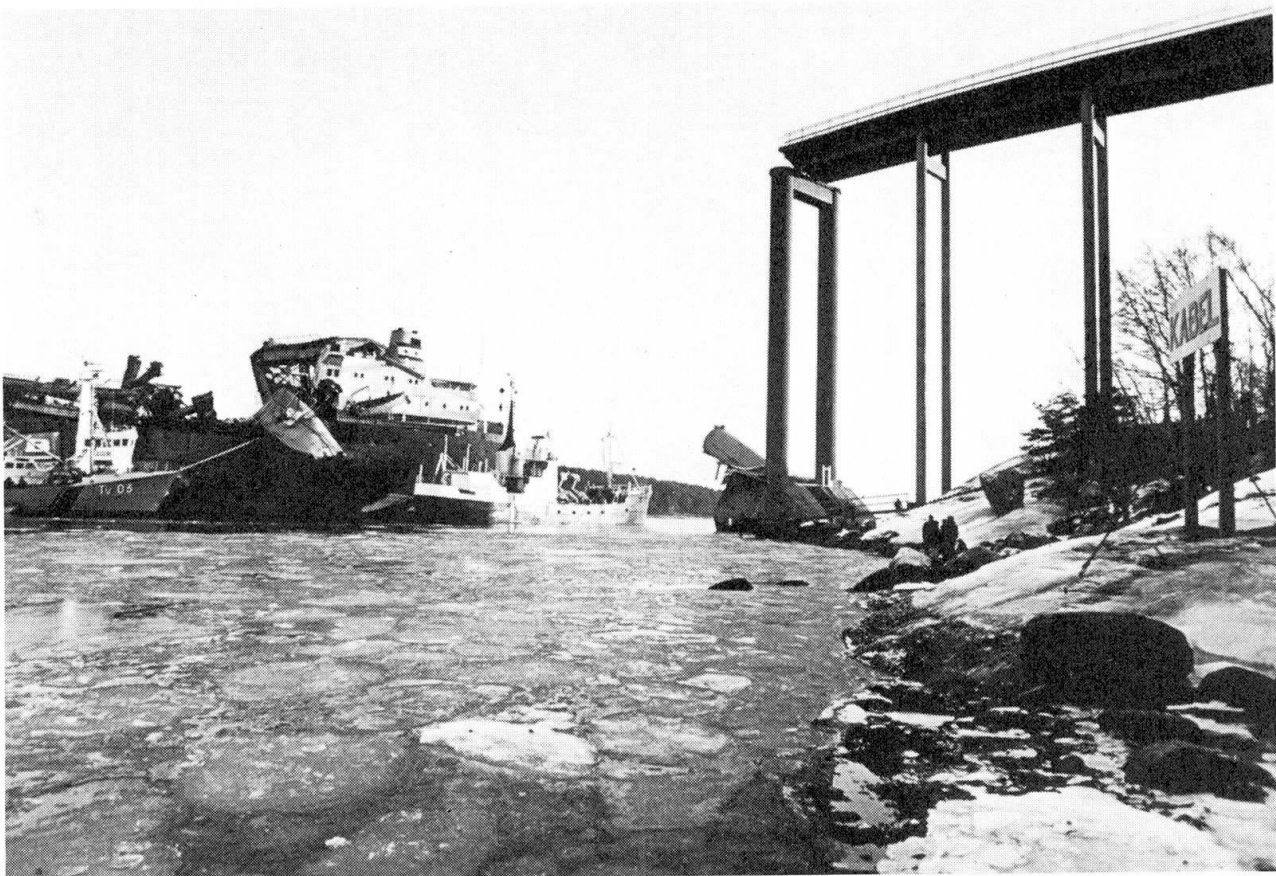
Almö-Bridge over the Askeröfjord, Sweden Hit on January 18, 1980, by a 15.000 t - freighter. 8 persons killed. Photo: Courtesy of Construction News, London, England
