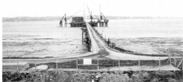
Construction of caissons at the end of the 500 m jetty.
