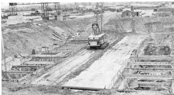
Excavation of the southern anchorage – strutting of longitudinal concrete walls.
