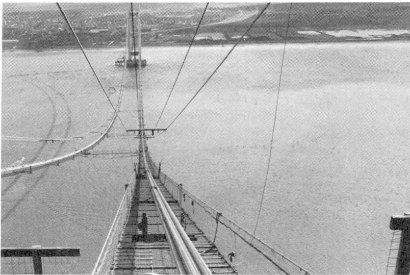
Mainspan cable part way trough spinning process.
