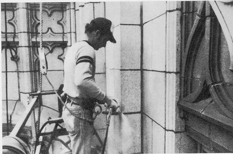
Fig. 7: Cutting of new expansion joints.
