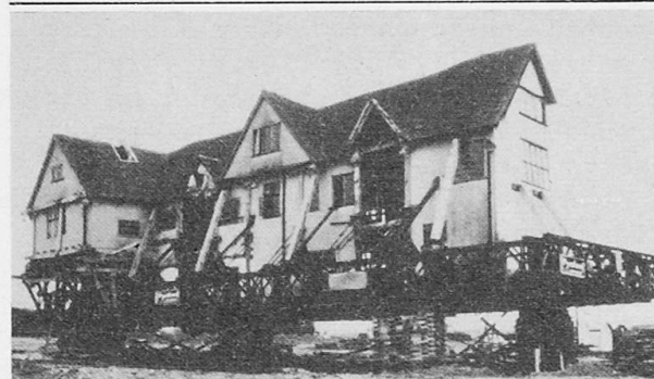
Fig.12. Steel frame under 17th Cent. mansion.
