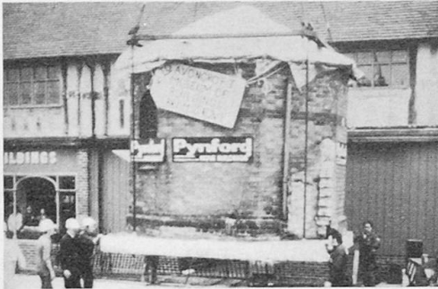
Fig.1. Crane lifting building.
