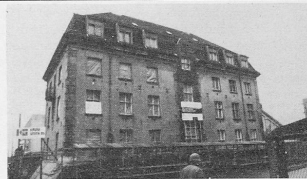
Fig.13. 2500 T being moved - Norway.
