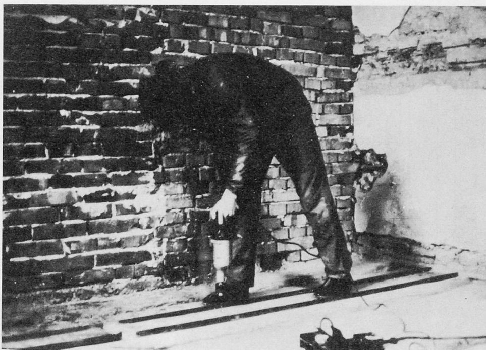
Fig. 6. Rough drilling with a drilling template
