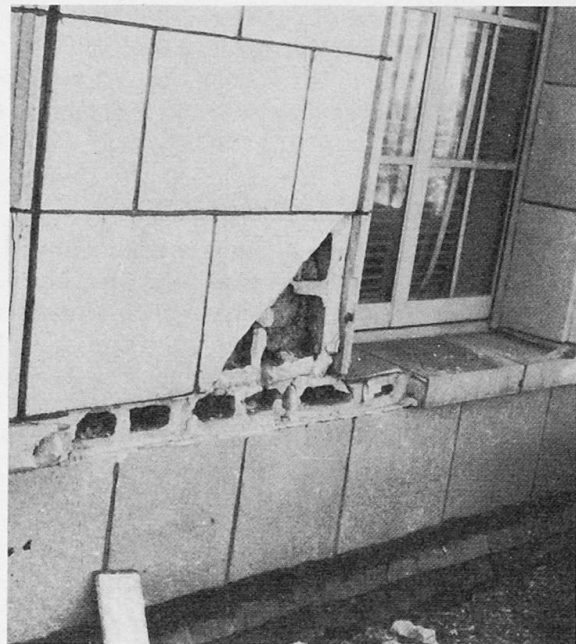
Fig. 4: Inspection opening
