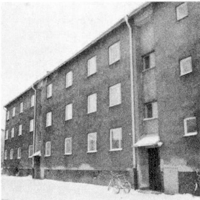
Fig. 1 Typical building from the fifties ready for renovation
