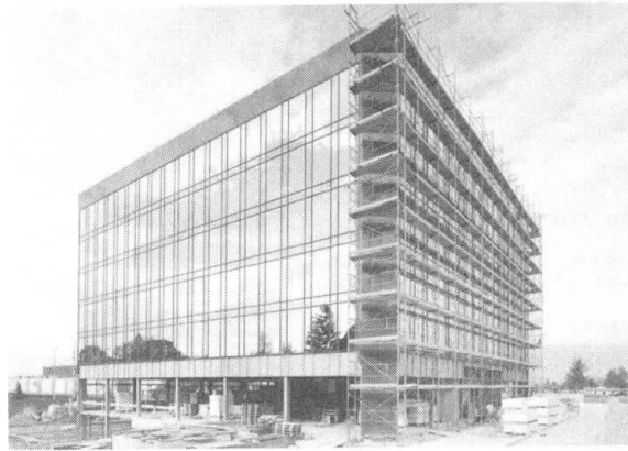
Fig 6 Building "Tour Balexert" at Geneva. All windows and curtain wall in "High Insulation Technology". No heating, only ventilation at 20-22°C.
