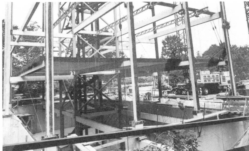
Fig. 9 Demo-building under construction
