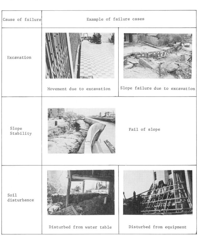
Fig. 1 (Cont.) Collapse cases of sub-structures
