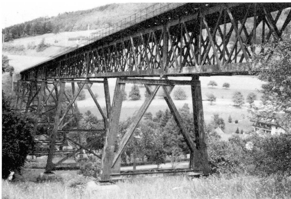
Fig. 2 Bridge of the "Museumsbahn"
