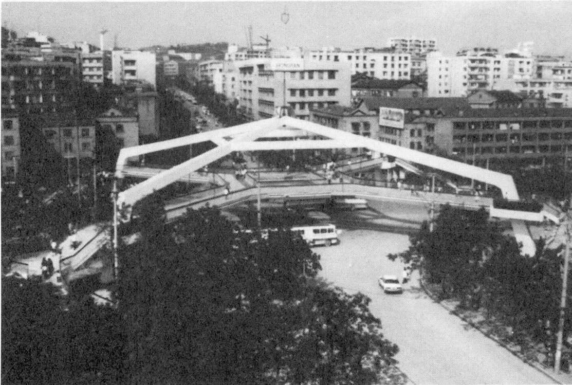
Fig. 3 Guanyinqiao Bridge in Service
