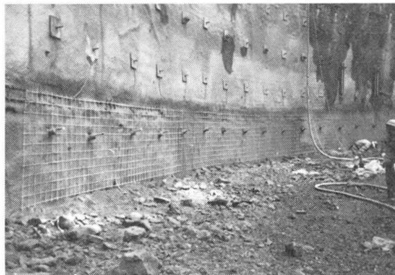
Fig. 2 Reinforcing grids for shotcrete
