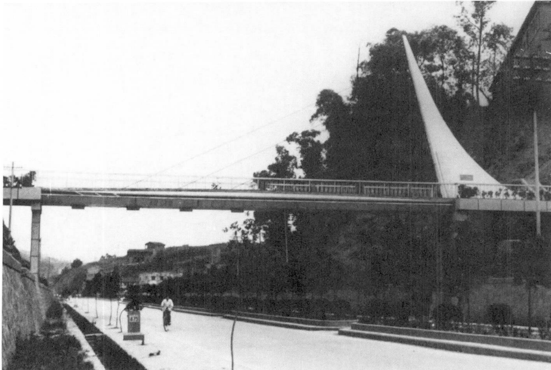
Fig. 1 GRP Pedestrian Cable Stayed Bridge
