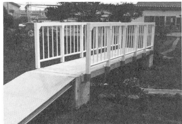
Fig. 11 Prestressed concrete pedestrian bridge
