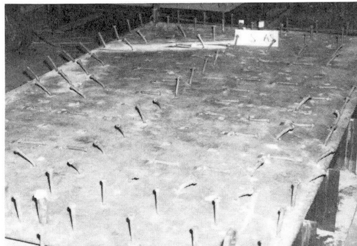
Fig.5 Typical shearing-off of studs(2A-2).
