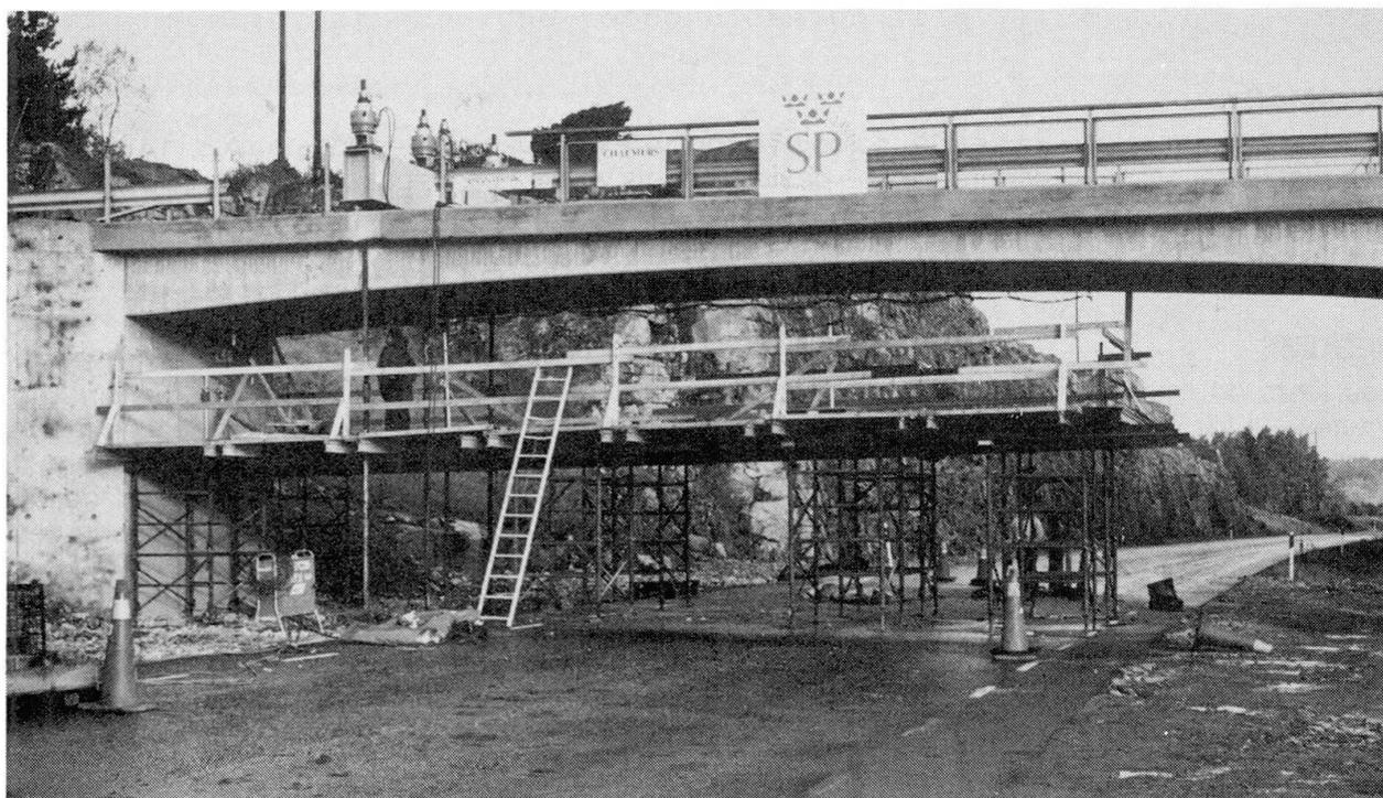
Fig. 1 Non-prestressed bridge during test preparation.
