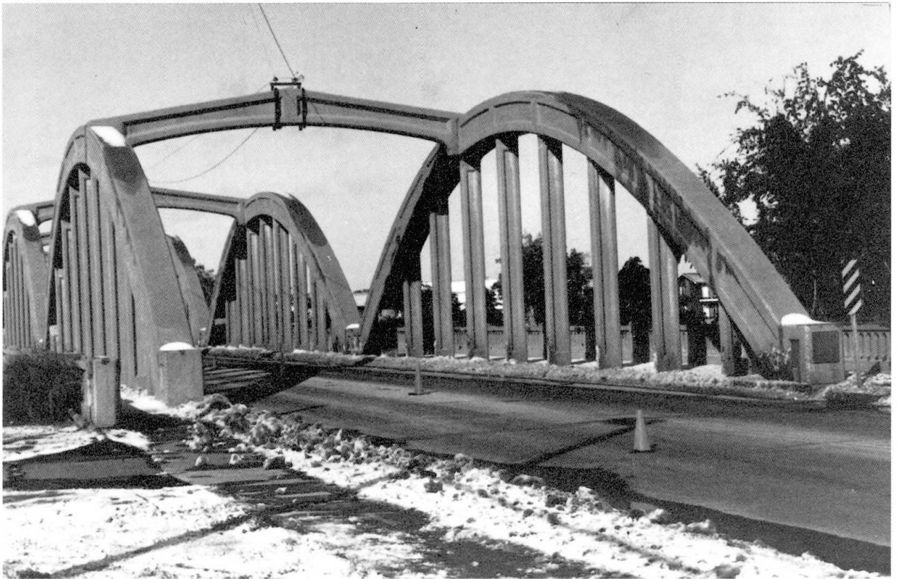
Figure 3. Circa 1930 patented Marsh encased steel through arch span at Wichita, Kansas.
