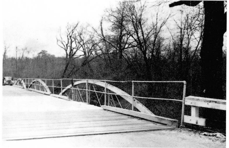
Figure 5. Ca. 1860 King bowstring truss bridge at Allenwood, NJ.
