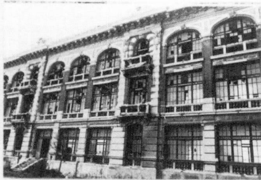
(a) Part of the Extension Building
