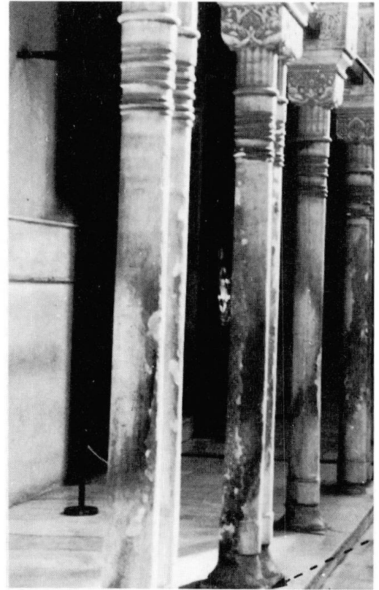
Fig. 3 Progressive reduction in height of bases, and damaged shafts according to mechanical weakness plane.
