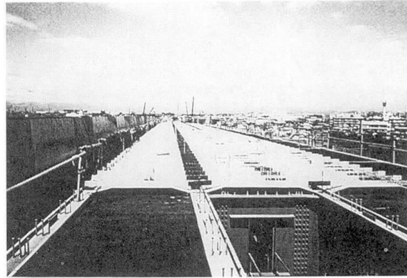
Fig.7 Setting of Bottom form on girders
