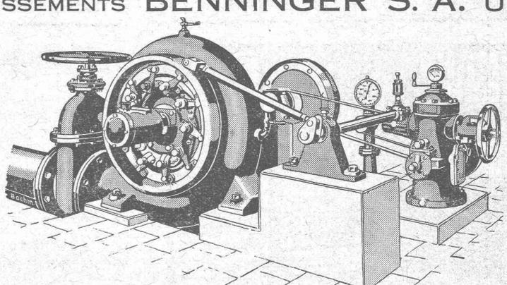
**TURBINES HYDRAULIQUES, RÉGULATEURS**
