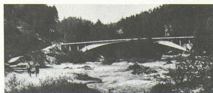
2051 Schwarzenburg 1932 Rossgrabenbrücke, Ing. Maillart Robert
