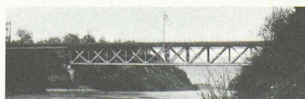
4080 Hagneck 1870–75 Brücke Hagneck, 55 m Länge, 5,5 m Breite, Ing. Thormann, Ott & Co
