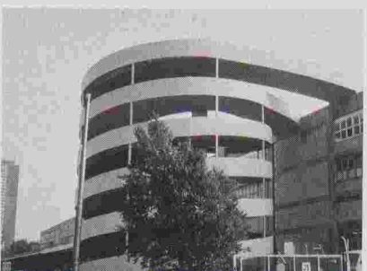
Rampe de parking Migros Herdern
