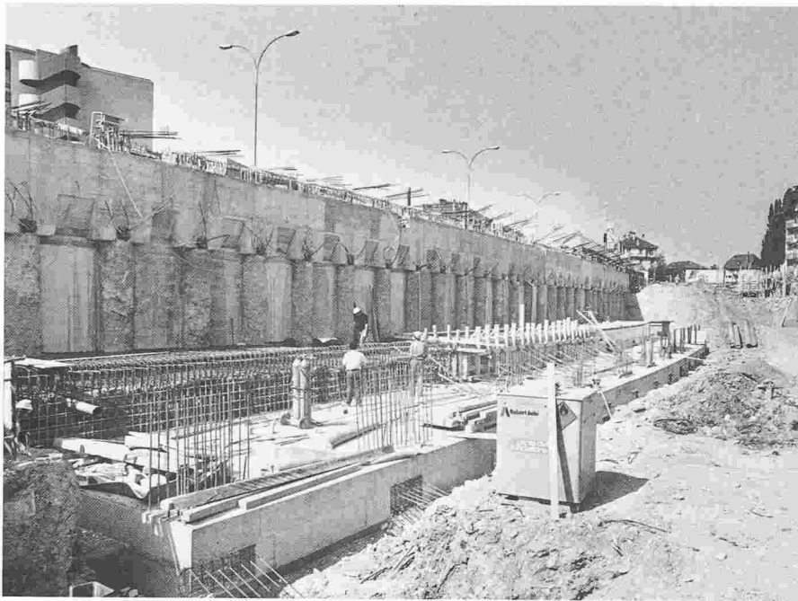
Fig. 15. – Station de Malley.
