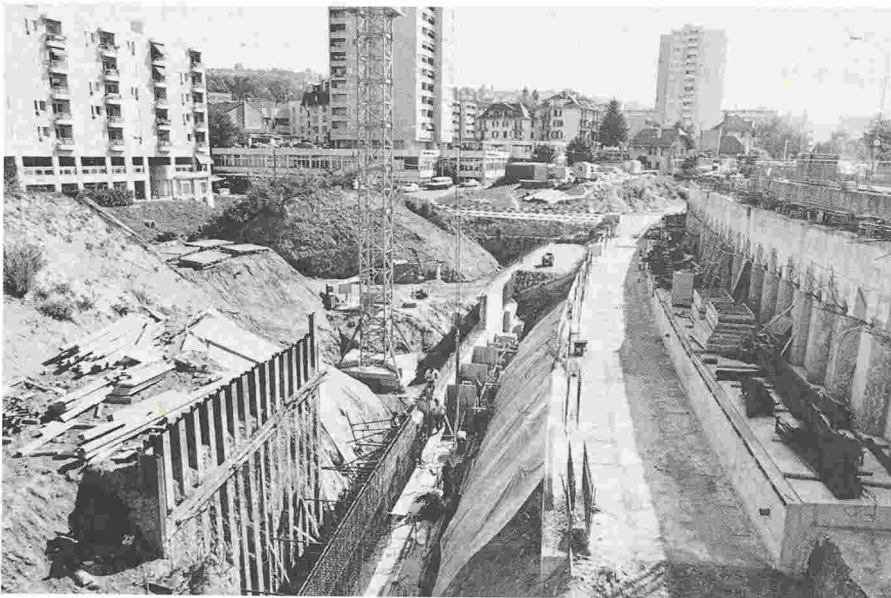
Fig. 16. – Station de Malley.
